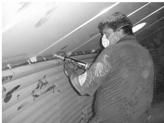
Fig. 10 Sealing the roof to wall joint
